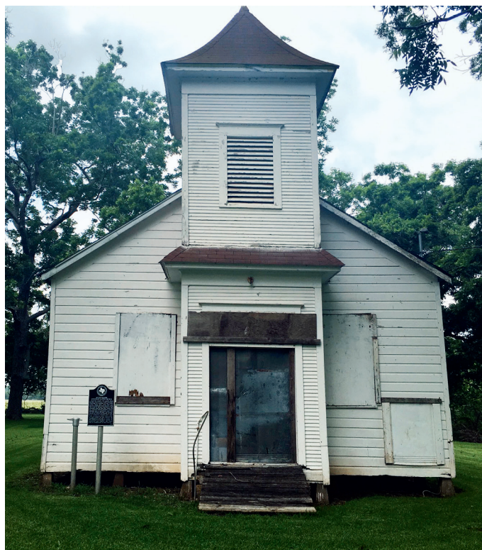
Mt. Pilgrim Missionary Baptist Church, Matagorda County, Texas. The church was built on land acquired around 1885 by men and women who were once enslaved. The building was a place of worship and a community school until around 1930.
